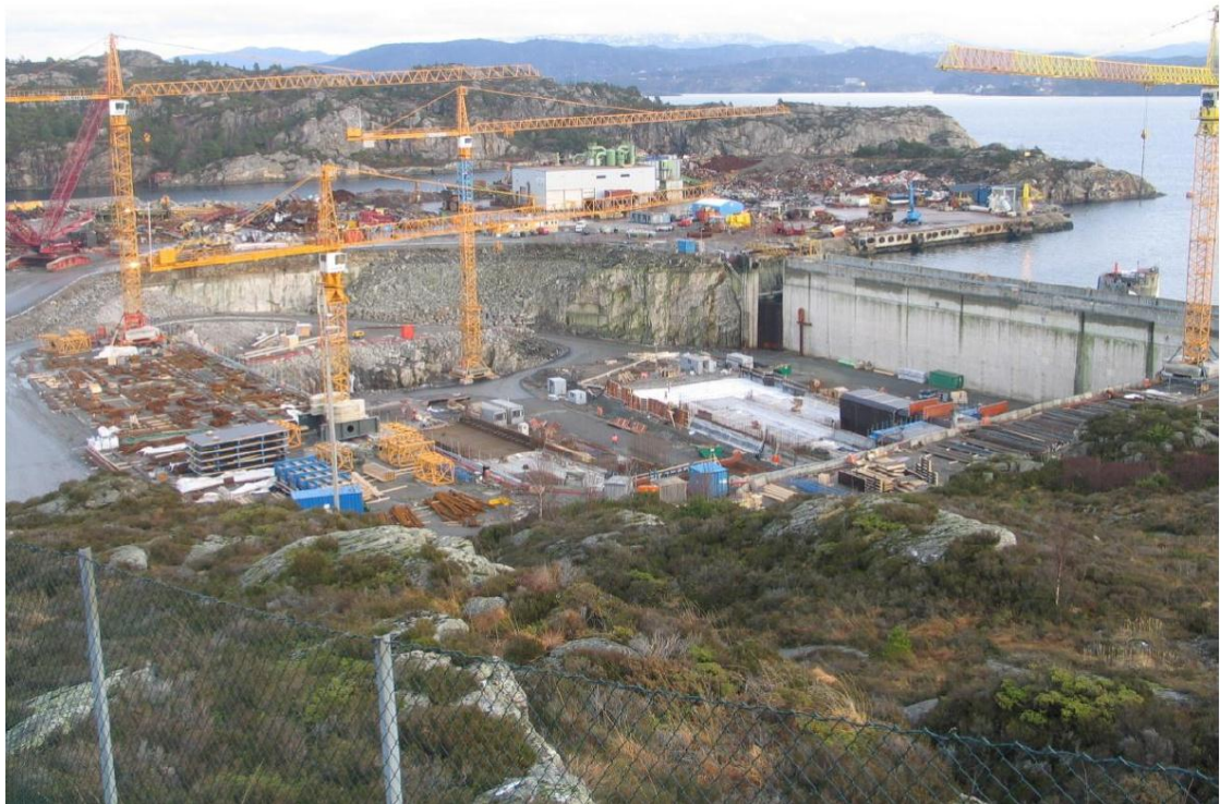
FIGURE 4-2 CONCRETE CAISSON IN A DRY DOCK
