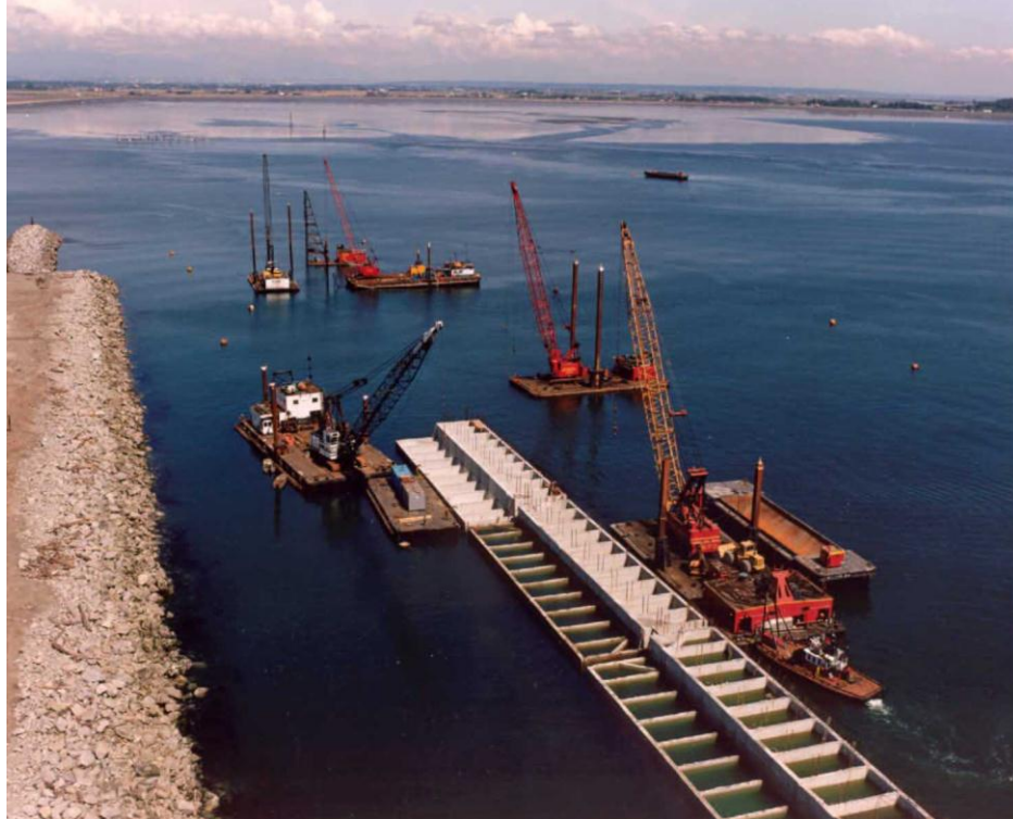
FIGURE 4-4 CONSTRUCTION OF A CONCRETE CAISSON WHARF AT DELTAPORT
